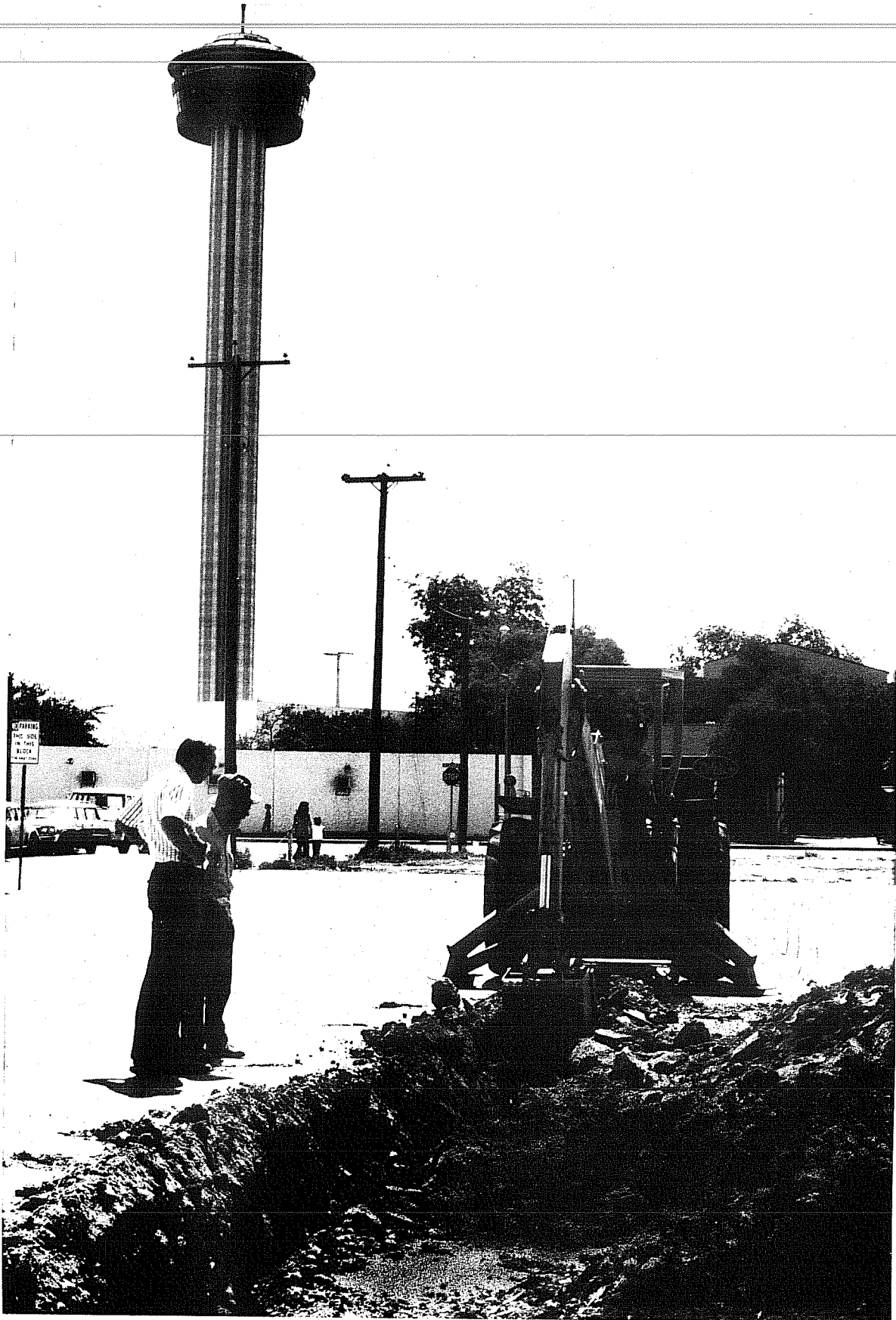
Figure 3. Trenching NCB 901. The parking lot (east portion of NCB 901), showing backhoe activity in progress, looking east toward Hemisfair Plaza.
