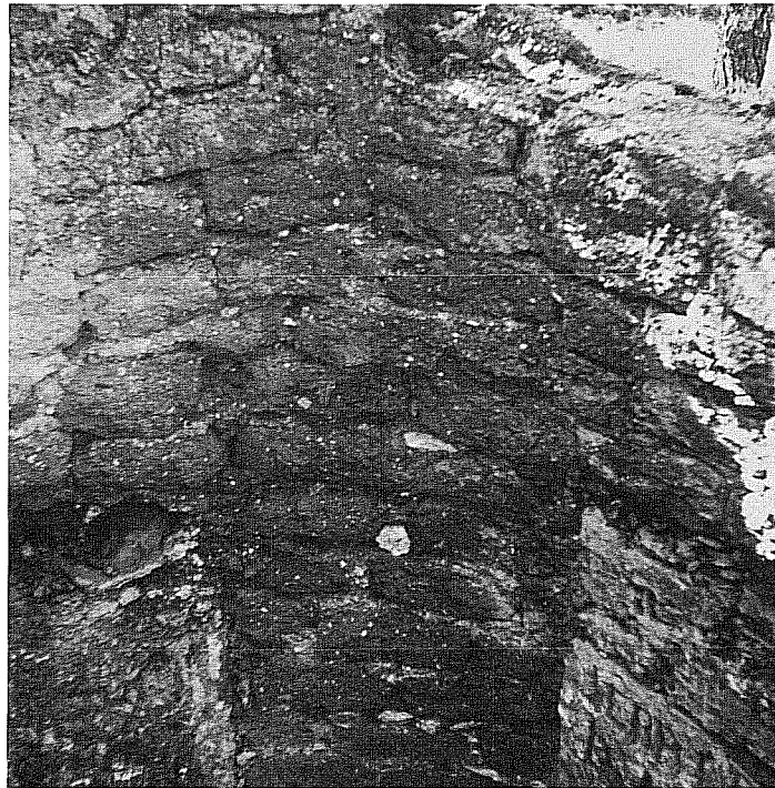
Figure 3. Lime Kiln on Olmos Creek (41 BX 367) . a, view of front of kiln from the creek bed, looking west; b, interior construction of the kiln, showing fired adobe brick set in sand and lime mortar.
